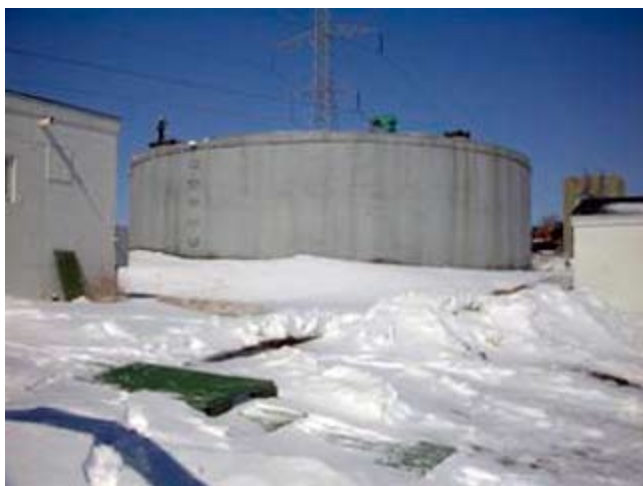
Figure 8 Continually stirred tank reactor (mixed digester)
