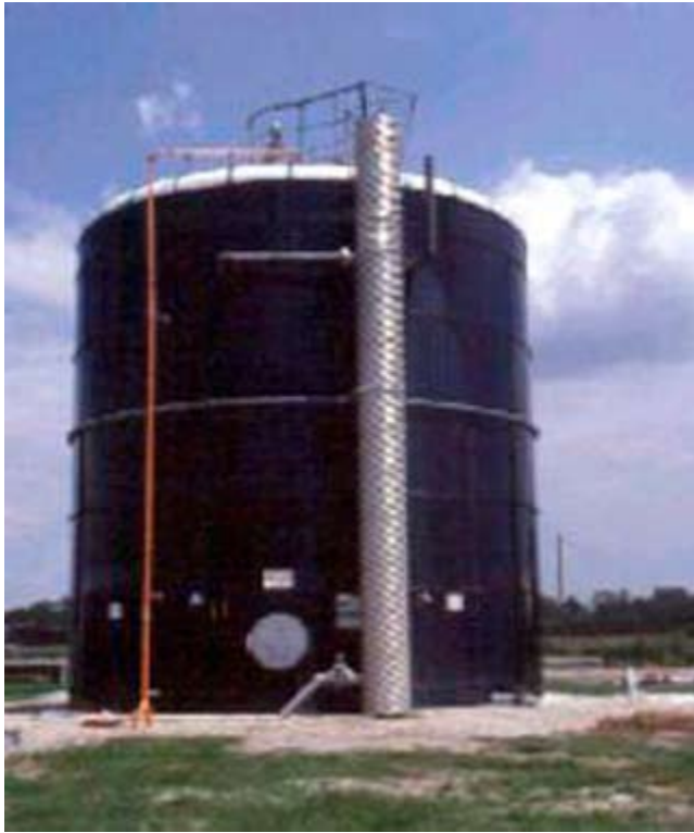
Figure 9 Fixed-film digester
