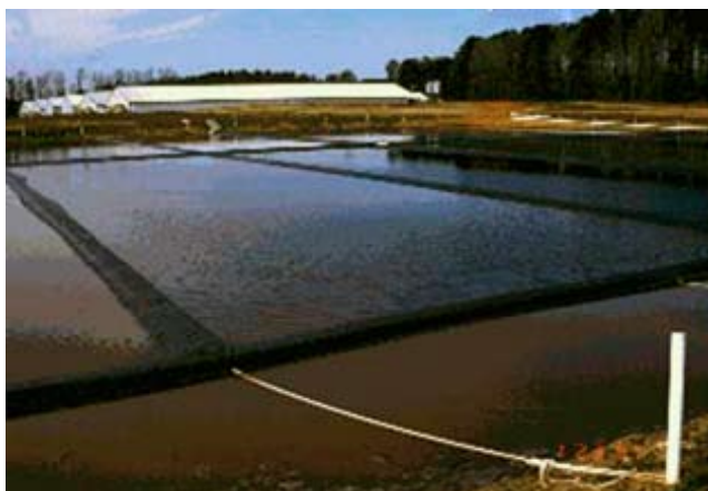
Figure 6 Partially covered anaerobic swine lagoon
